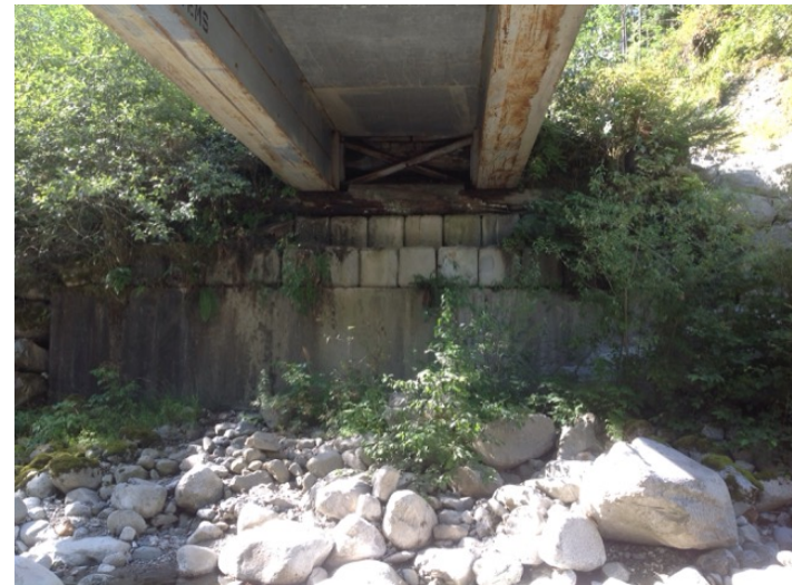
Right Bank Abutment when facing downstream
