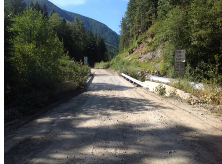
Approach from Left Bank when facing downstream
